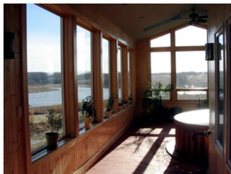
Smart use of window design and placement can add ambiance and reduce utility costs.
