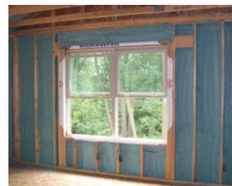
Closed-cell insulation significantly increases the "R" factor.
